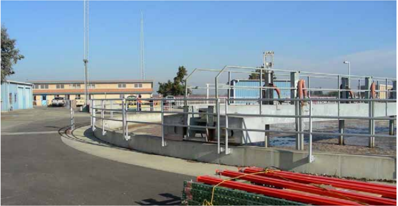
Wastewater Treatment plant facilities, looking north.
