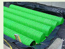
Triton stormwater chambers are a typical semi-circular linked chamber system.
