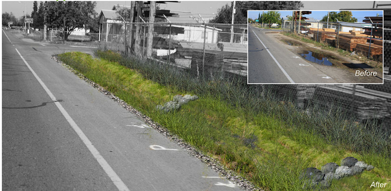
Vegetated swales, such as this installed in a parking lot, can both treat and convey runoff, eliminating the need for some catch basins and pipes.
