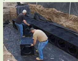
Cudo Cubes are an example of a typical modular block system.
