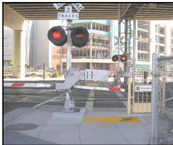
Pedestrian Gate Arm, Emergency Exit Gate and Adjacent Fencing 19
